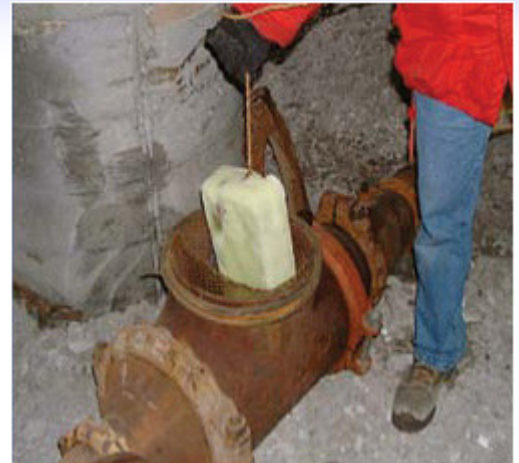
Floc Log ® placement in a pipe system
